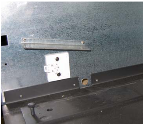
Fit the cable with female connector for ES 904 through the hole in the cassette.
